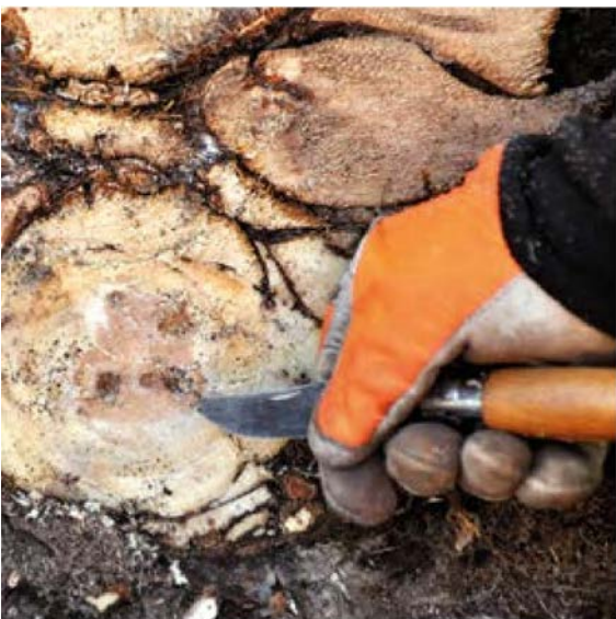
Figure 60. Inspected the cutting area with knife to check the depth of the infestation
