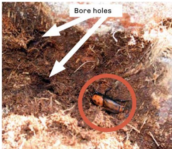
Figure 10. Damage with holes (white arrows) and an adult near the holes trying to enter (yellow circle)
