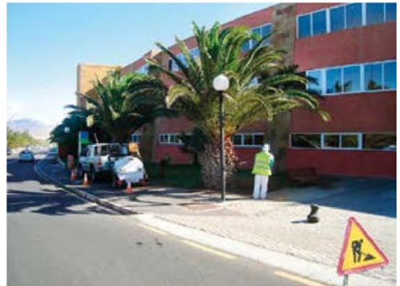
Figure 84. Preventive chemical treatment against RPW in an urban area
